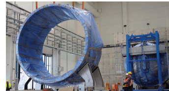
Installation of SPIDER Vacuum Vessel.
