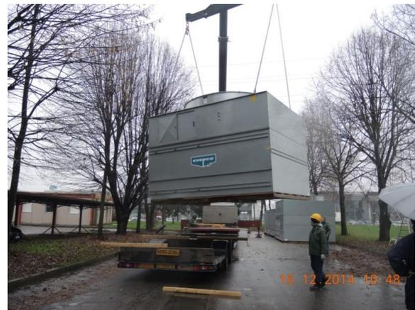
*Fig. 4.9: Delivery of Cooling Towers at CNR Research Area, to be then installed on the roof of PRIMA Buildings*
