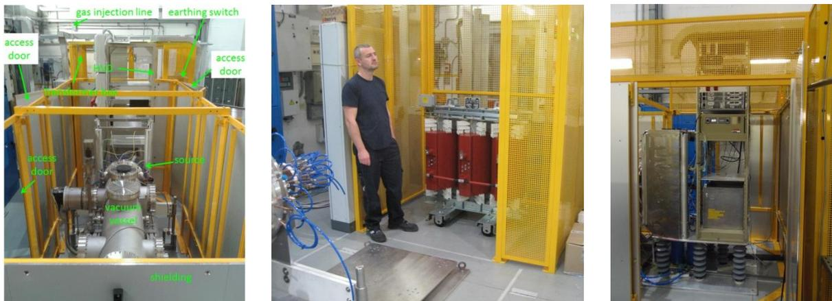
Fig. 4.53: left: X-ray shield after installation; centre: insulation transformer; right: high voltage deck
