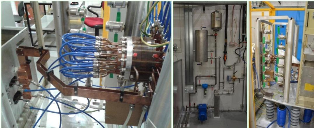
Fig. 4.54: left: RF transmission line; centre and right: components of the cooling system
