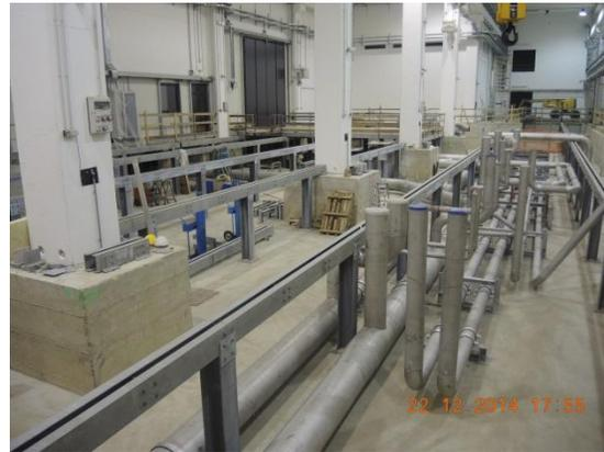
*Fig. 4.8: Cooling pipes installation inside Building 2 at level -2.0 m*
