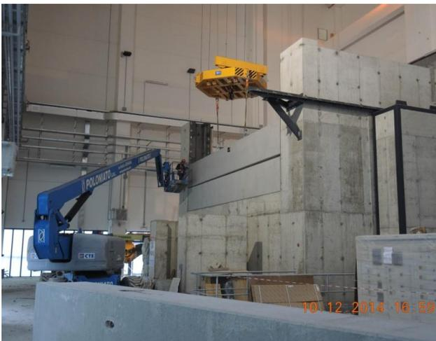
*Fig. 4.2: SPIDER bio-shield: installation of the removable concrete beams*
