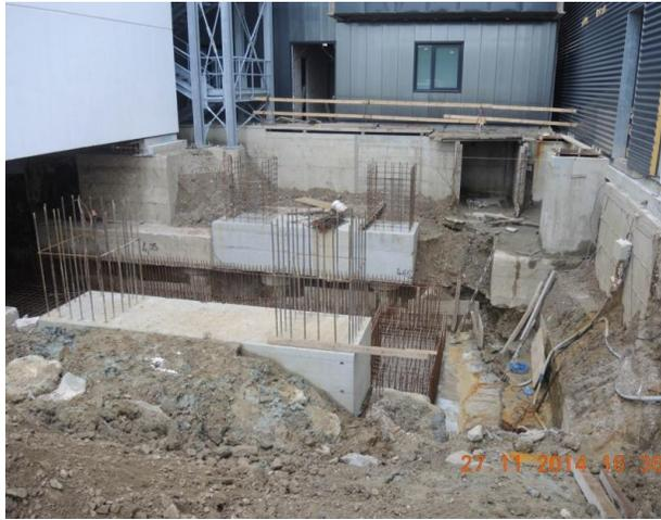
*Fig. 4.4: Concrete basement of the TL2 tower*
