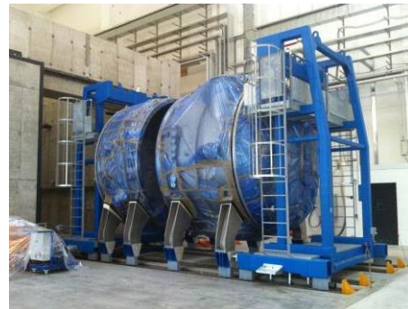
Fig. 2.1.14: Assembly on-site of SPIDER VV
