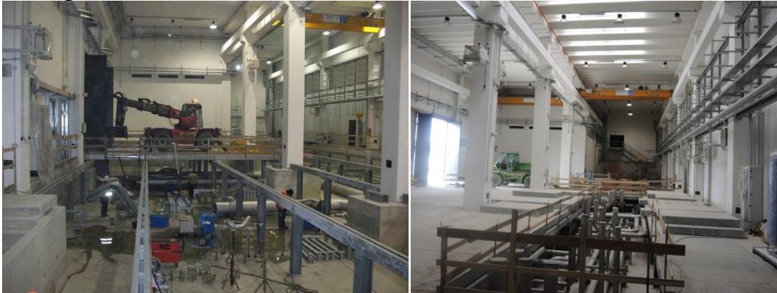
Fig. 2.1.10: Cooling pipes installation inside Building 2 at level -2.0 m; the floor at ground level is ready for next installation of pumps and heat exchangers
