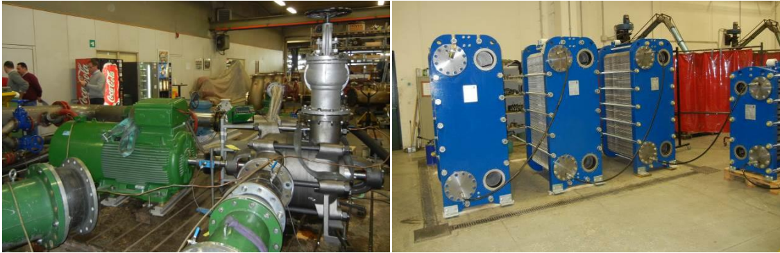
Fig. 2.1.8: Pumps (Garbarino) and Heat Exchangers (Sondex) for primary and secondary circuits during factory tests
