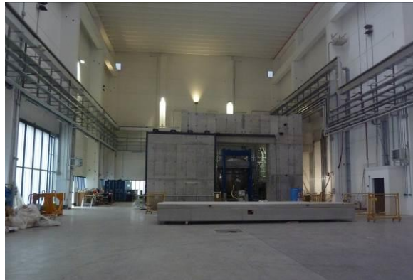
Fig. 2.1.3: PRIMA Site: view of the SPIDER bio-shield inside building 1 complete of removable concrete beams
