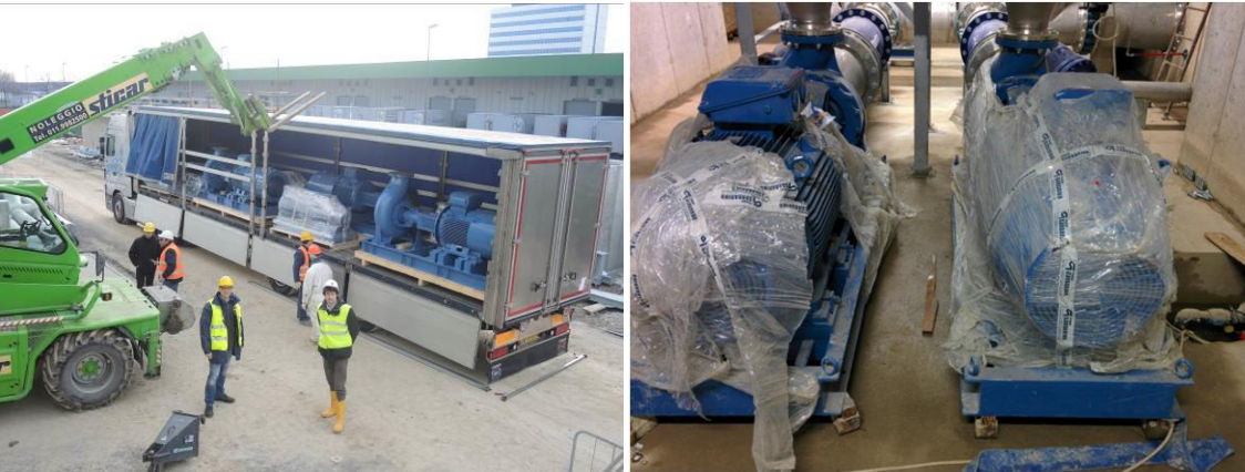
Fig. 2.1.9: Unloading and installation of pumps of tertiary and secondary circuits in Building 2 at level -4.0 m
