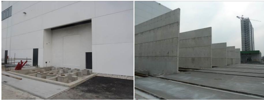
Fig. 2.1.5: area hosting MITICA PS. right: 1MV insulating transformer pit; left: DCG pits
