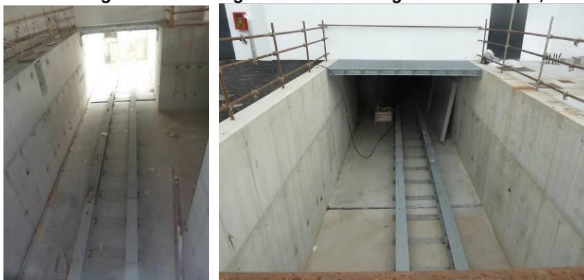
Fig. 2.1.6: PRIMA Site: view of the pit crossing building 8 and hosting part of the MITICA TL. Note the still beams to be used to anchor the TL post-insulators
