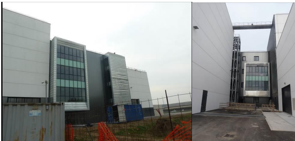
Fig. 2.1.2: front and rear view of building 12 hosting SPIDER/ MITICA control rooms
