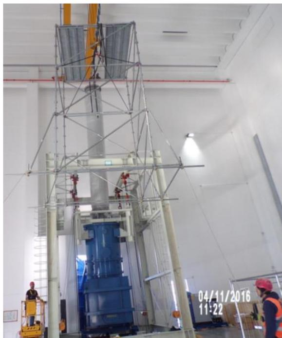
**Fig. 2.1.39 High Voltage *Bushing of the -1MV Insulating Transformer***
