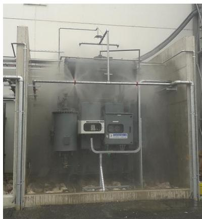
**Fig. 2.1.14 Test of fire-suppression system**
