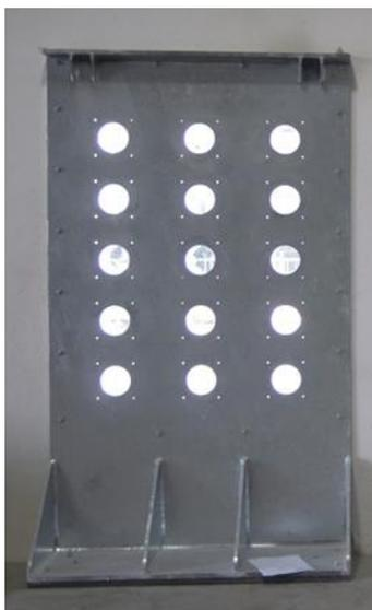
**Fig. 2.1.12 Supporting structure for AGPS cable feedthroughs**
