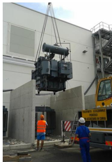
**Fig. 2.1.13 Placement of transformers in the pits**
