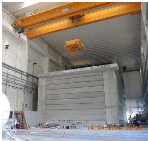
**Fig. 2.1.43 - Installation of a concrete slab of the MITICA bio-shield roof**
