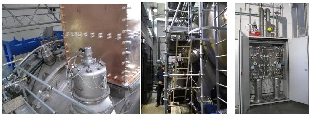
**Fig. 2.1.46 SPIDER GVS components: pumping system inside the bioshield (left, middle) and gas injection cabinet GIS-A (right).**
