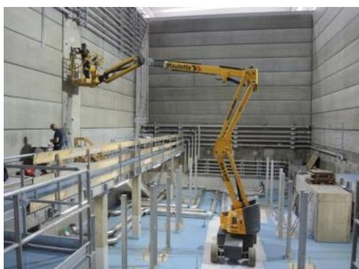
**Fig. 2.1.5 Installation of cooling pipes inside the MITICA Neutron Shield**
