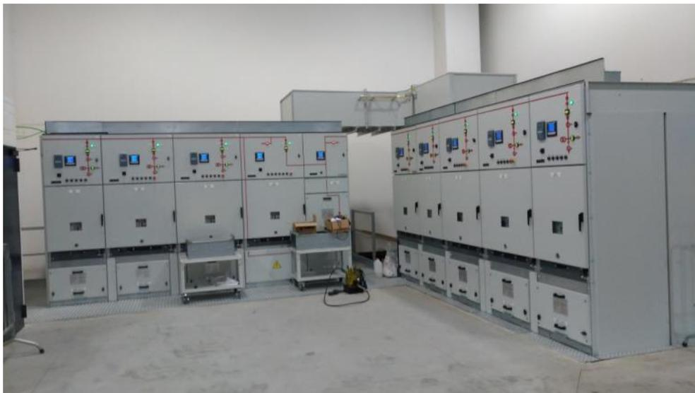
Fig. 2.1.7 – MITICA MV Distribution Board
