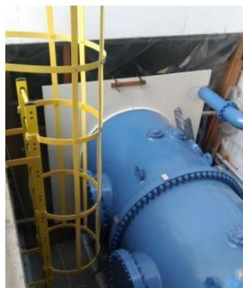
**Fig. 2.1.2 Special sealed and insulating closures of the MITICA HV Transmission Line**
