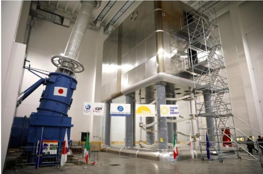
**Fig. 2.1.40 Overview of the HV components inside High Voltage All. On left: 1MV bushing of insulating transformer. On right: HVD1 with temporary scaffolding necessary to access inside the Faraday cage.**
