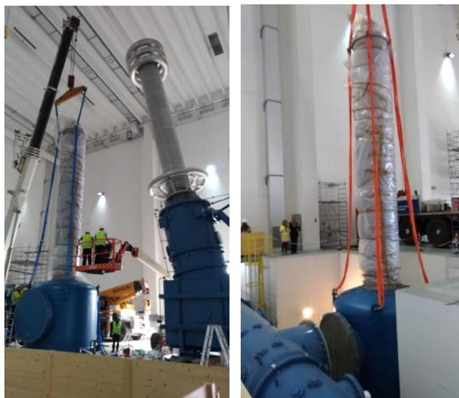
**Fig. 2.1.39 Installation of the HVBA inside the TL2 pit. Left: lifting of the HVBA before downloading in the pit. Right: HVBA inside pit with view of flanges interfacing the Connecting Piece**
