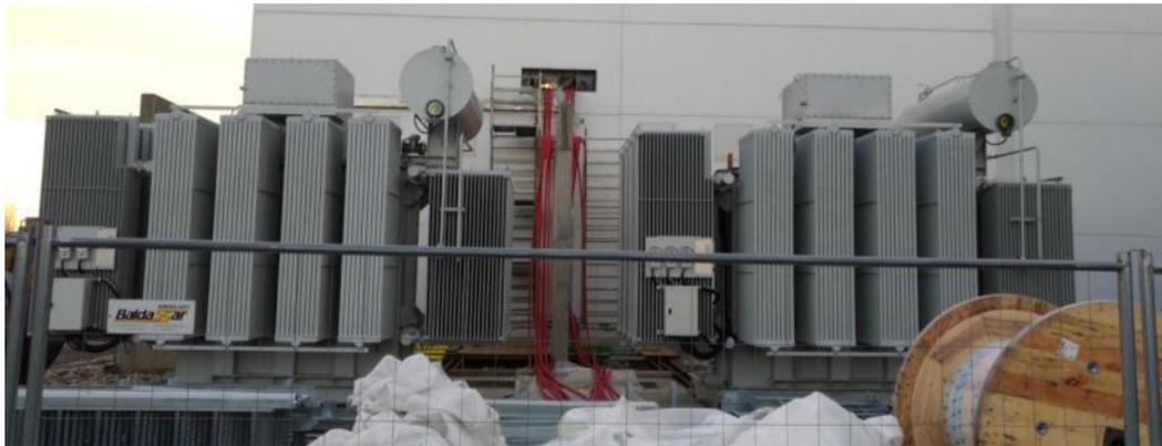
**Fig. 2.1.36 Step-down transformers**
