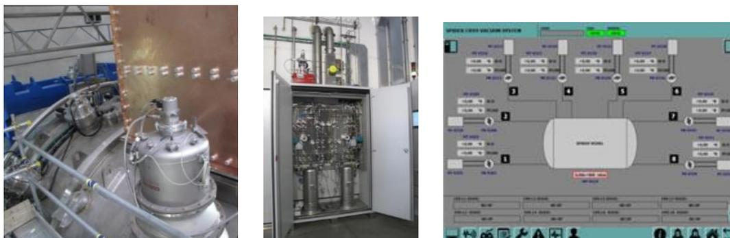
**Fig. 2.1.6 SPIDER GVS: pumping system inside the bioshield (left), gas injection cabinet GIS-A (middle), cryo control system HMI window (right).**
