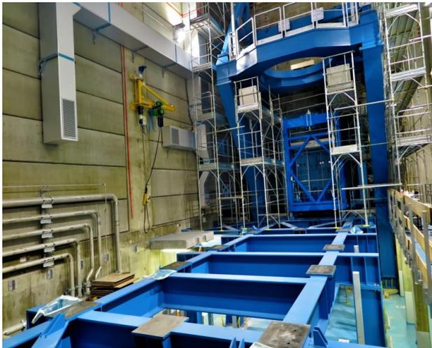
**Fig. 2.1.30** Picture of the MITICA Vacuum Vessel Support structure as finally assembled inside the MITICA Neutron Shield.
