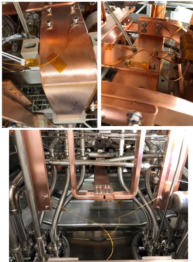
**Fig. 2.13 Installation of the new PG bus bars**
