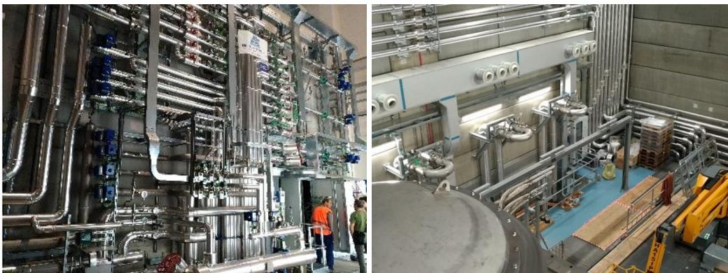
**Fig. 2.2 Left: Overall view of SPIDER distribution circuits on the back wall of SPIDER Neutron Shield; Right: Overall view of Primary Circuits pipes inside MITICA Neutron Shield**
