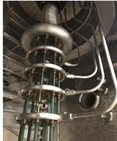
**Fig. 2.37 AGPS Short Circuiting Device (SCD) installed inside BSV**
