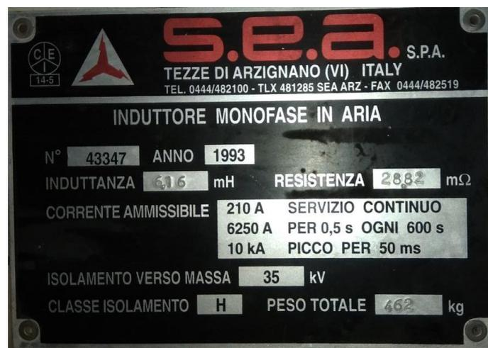
Figure 4-1 – plate data of the inductors that can be made available by the CRFX
