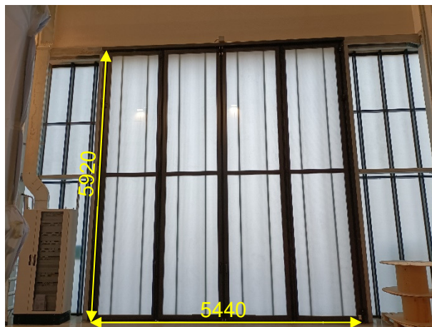
Fig. 4 - Building 1: material entry door A.
