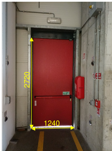
Fig. 3 - Building 1: pedestrian door n°6.
