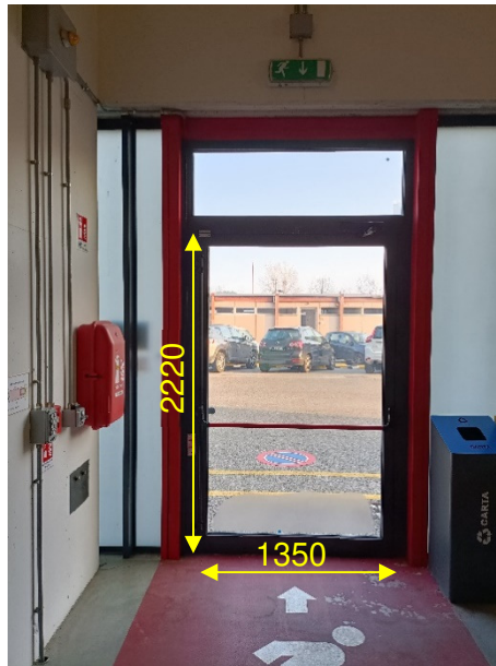
Fig. 2 - Building 1: pedestrian door n°2.
